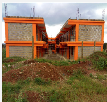
Figure 8a: Hostel on a Subdivided Land
